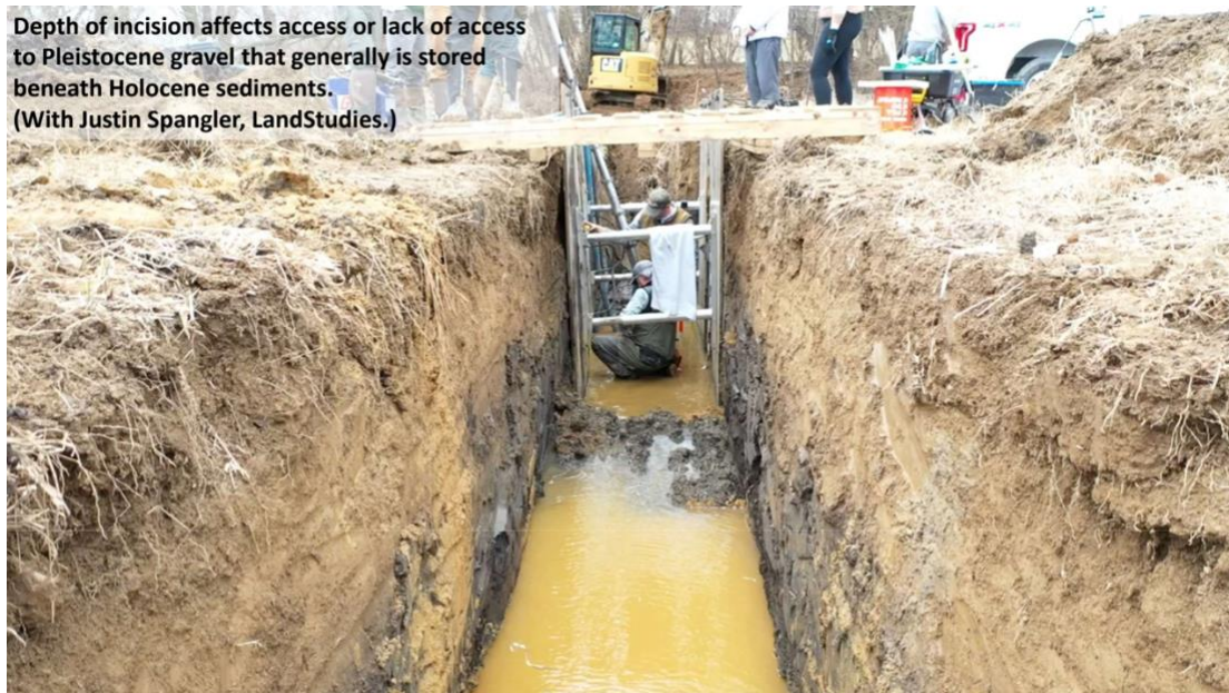
Figure 2. Images from Little Conestoga Creek in February 2023 during a restorative effort to rejuvenate about 2.5 miles of the impaired channel. Depth of incision affects access to Pleistocene gravel that generally is stored beneath Holocene sediments. (With Justin Spangler, LandStudies.)
